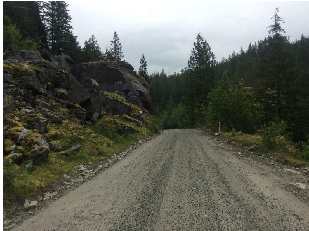
Photo 8 ~3.9 km Chehalis FSR, narrow road section with talus rock slope above
