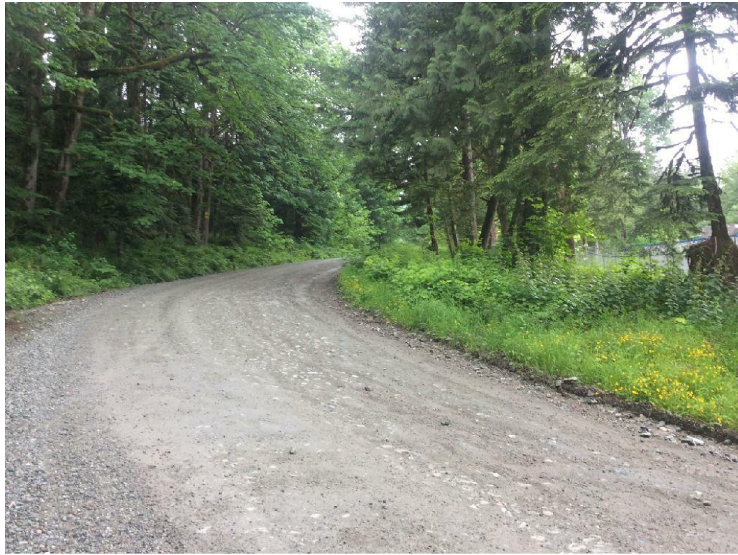
Photo 5 1.5 km Chehalis FSR, road section with washboard surface
