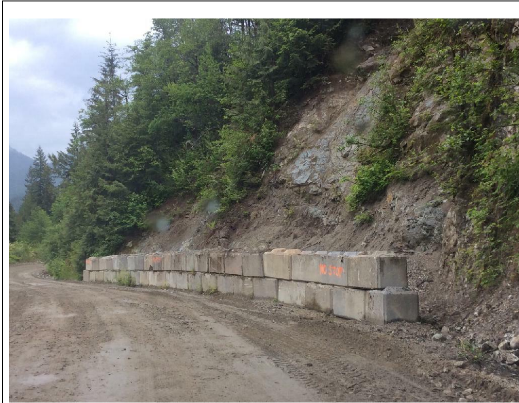
Photo 14 10.1 km Chehalis FSR, rock fall catchment retaining wall
