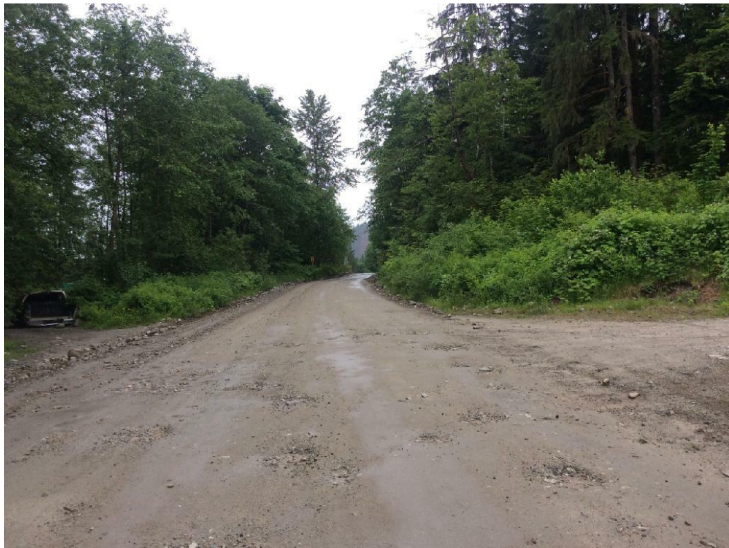
Photo 10 5.8 km Chehalis FSR, wide road with existing pullouts / junctions
