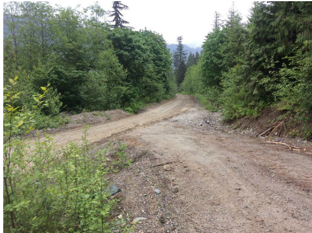
Photo 18 11.5 km Chehalis FSR, view from existing gate towards FSR
