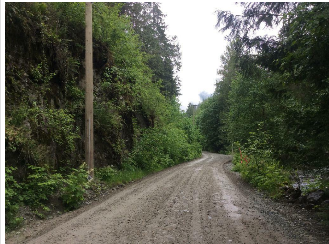
Photo 2 Narrow road section at 0.6 km.
