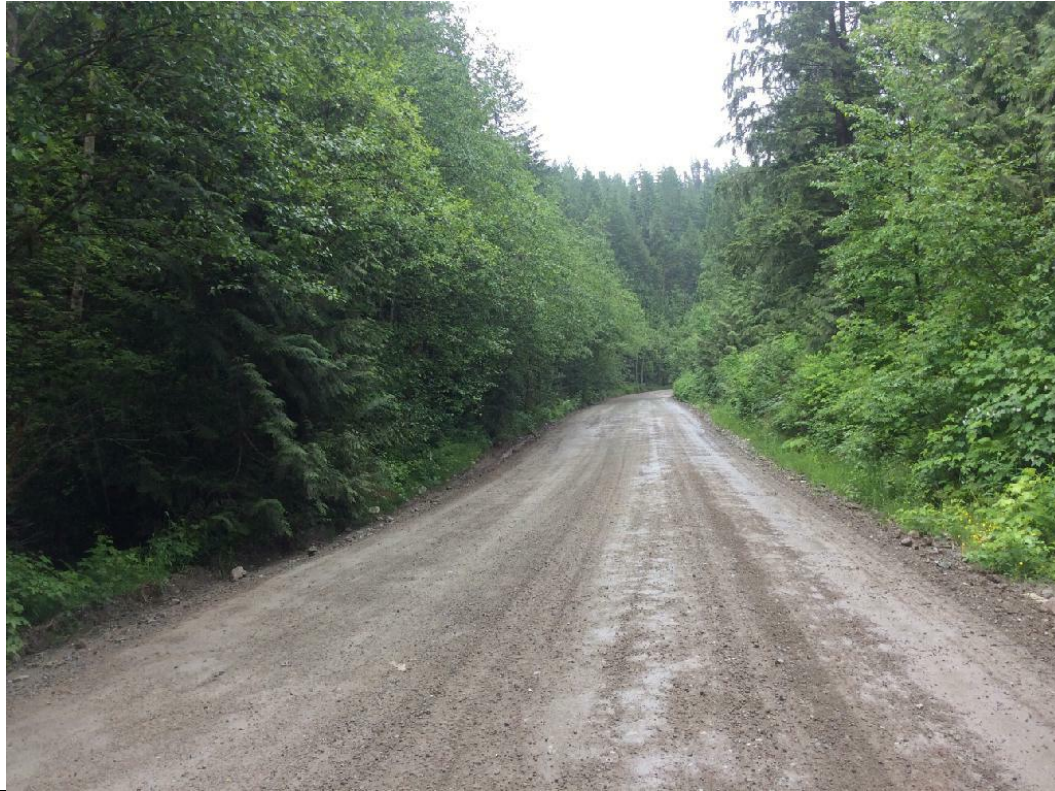
Photo 9 4.4 km Chehalis FSR, typical 7-8 m road width
