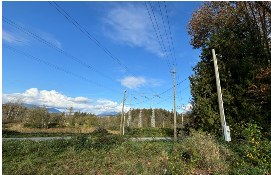
Figure 6: On-site visit photograph of hydro corridor.
