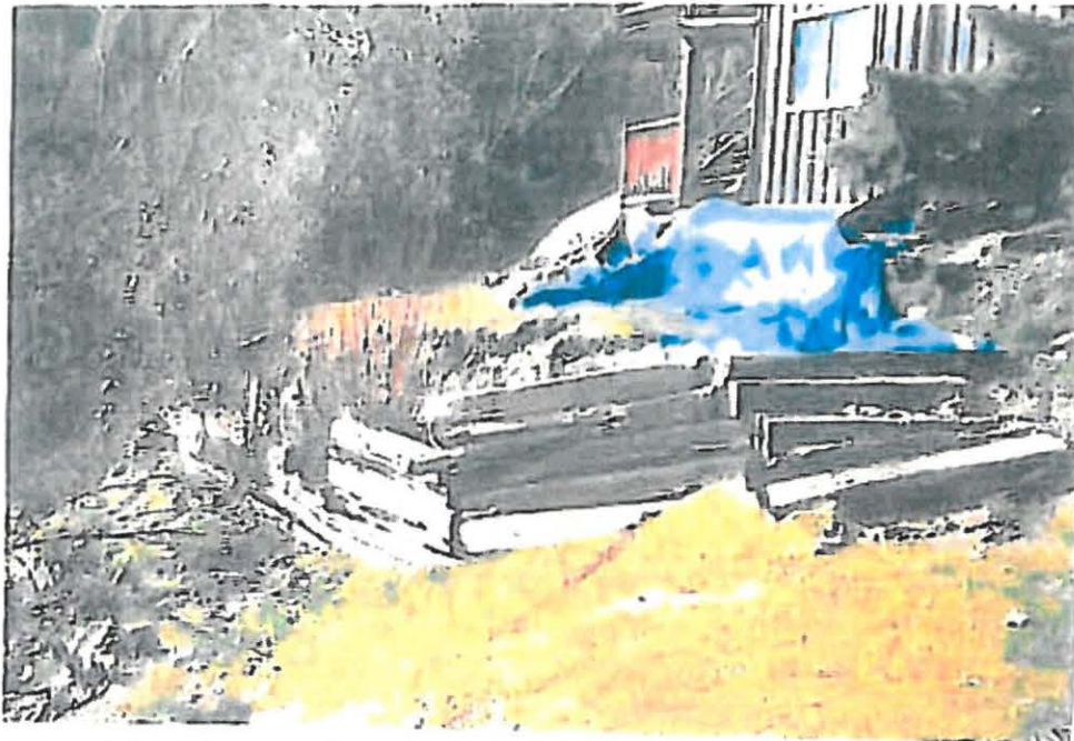
Photo 1. View WNW showing slide below MacGregor house at 4164 Thor Road. Note the sheared soil mass in the foreground.
