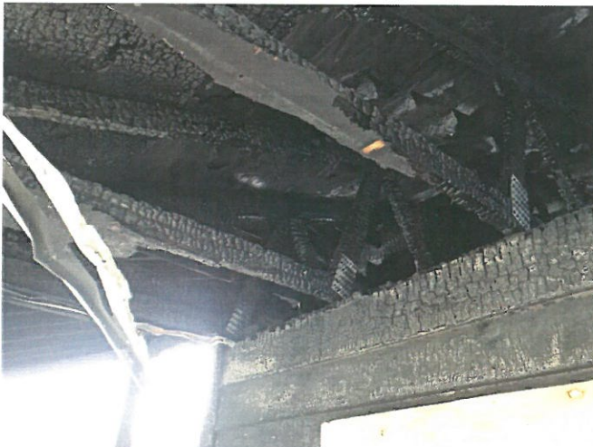
Photo 5: Roof and Wall damage over back deck/walkway
