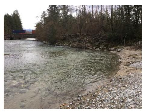
Photo 9 Looking downstream at the armoured Norrish Creek Dyke 80 m upstream from the CP Railway Bridge where the dyke transitions from a river dyke to a setback dyke. The  $D_{50}$  of the riprap is 600 mm.
