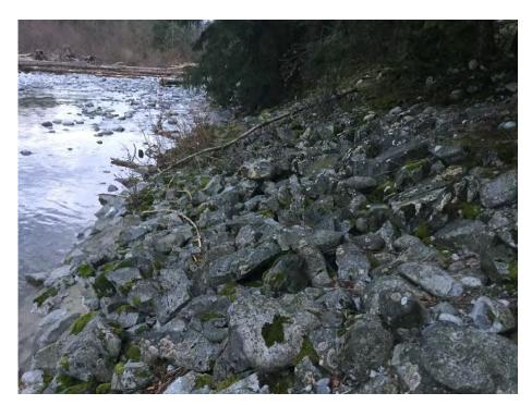
Photo 13 Looking downstream at the armoured Norrish Creek Dyke 250 m downstream of the fan apex. The  $D_{50}$  of the riprap is 300 mm.
