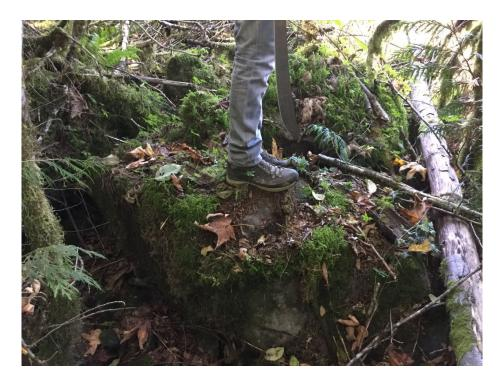
Photo 21 The toe of the bank was armoured with large angular boulders that were covered with moss and vegetation. Many of the larger boulders average 1 m or greater in diameter.
