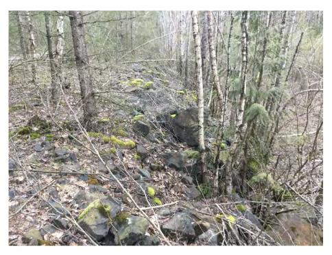
Photo 12 Norrish Creek Dyke along a typical armoured setback portion. Photo is just downstream of the upstream limit of continuous armouring 680 m from the CP Railway Bridge. The height of the dyke is approximately 2 m above the creek side floodplain. The  $D_{50}$  of the riprap is 500 mm.
