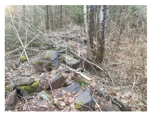
Photo 10 Norrish Creek Dyke along a typical armoured setback portion. Photo is 100 m upstream of the CP Railway Bridge. The height of dyke is approximately 2 m above the creek side floodplain. The  $D_{50}$  of the riprap is 500 mm.
