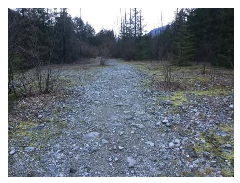
Photo 15 Looking downstream at the 20 m wide Norrish Creek Dyke crest adjacent to the eroding bank section.
