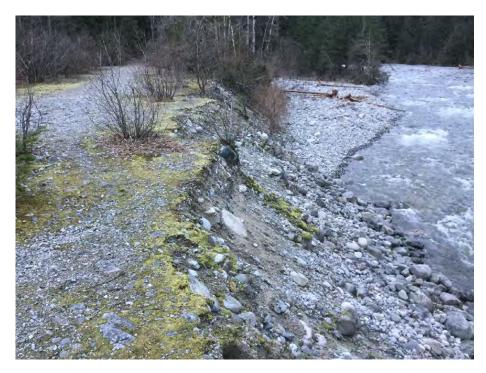
Photo 14 Norrish Creek Dyke along the 25 m long eroded bank section which is located 130 m downstream of the fan apex. The bank is approximately 3 m high.
