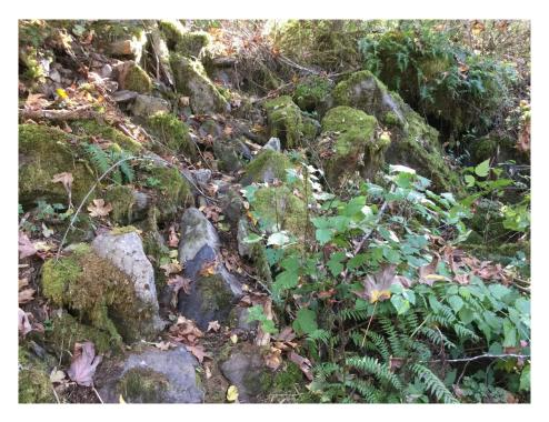
Photo 34 The armoured bank averages 3 m high and all of the rock appears to be angular quarried rock.
