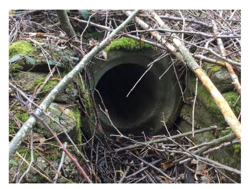
Photo 5 450 mm diameter concrete culvert inlet at the southwest corner of the Subject Property. The invert of the inlet is the lowest point on the property at 6.35 m GD.
