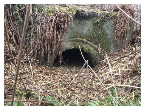
Photo 7 500 mm diameter concrete culvert outlet under the CP Railway adjacent to the middle of the Subject Property. The inlet could not be located and there was no evidence of past flow in the pipe.
