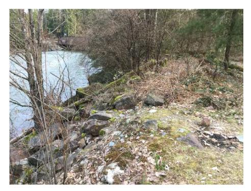
Photo 8 Looking downstream from the crest of the armoured Norrish Creek Dyke 80 m upstream from the CP Railway Bridge. The D<sub>50</sub> of the riprap is 600 mm.
