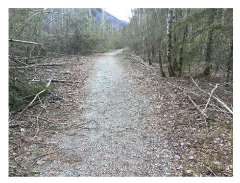
Photo 11 Typical view of the crest of the Norrish Creek Dyke. The crest averages 8 to 12 m wide but is up to 20 m wide at the upstream end where the dyke is not armoured.
