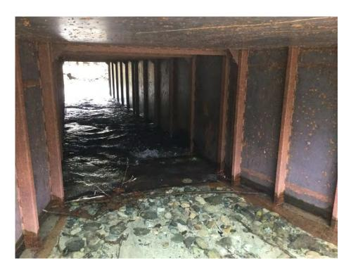
Photo 6 Looking downstream on Inch Creek at the inlet of the steel box culvert under the CP Railway. The culvert has a span of 2000 mm and a height of 1600 mm.
