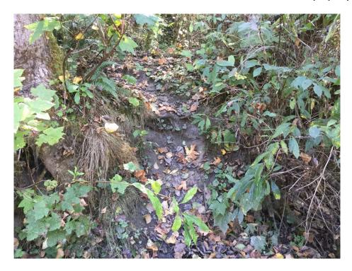
Photo 44 The bank at the downstream end of the property does not appear to be armoured .The exposed bank material is predominately fine grained.
