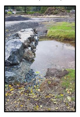
The three culverts resulted in the destabilization of the stream channel, loss of flow in Spring Creek and impacted fish passage.
