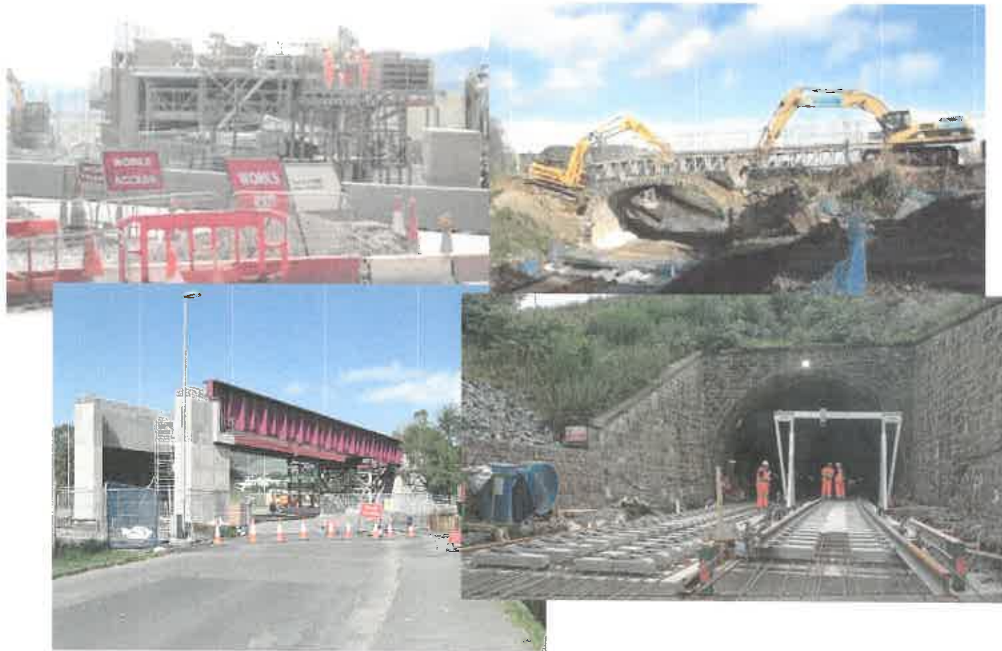
New Bridges & Refurbished Tunnels
