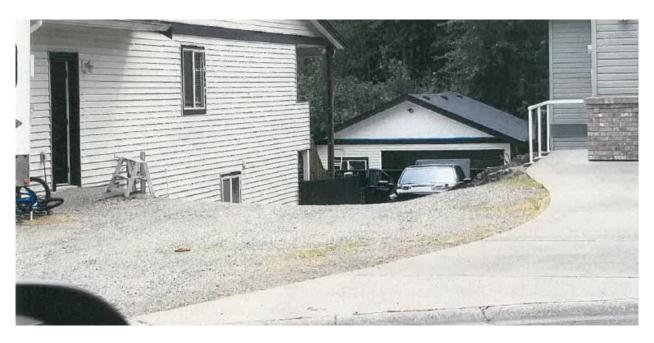
Image of the constructed shop from Berston Road (August 12, 2020). Covenant BT217825 requires floor area to be 0.4 metres above Berston Road. The shop does not meet this requirement
