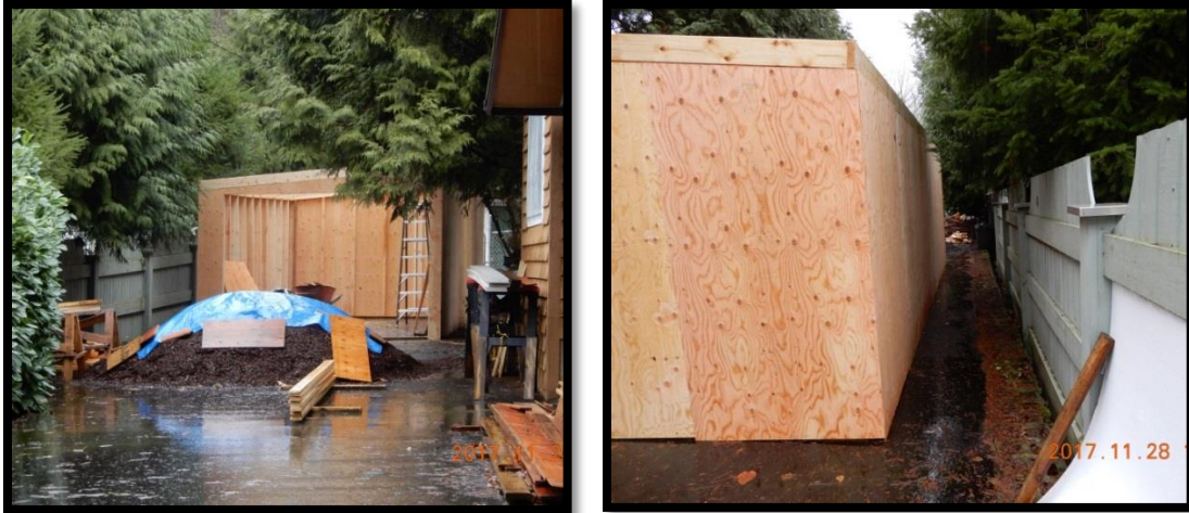
Photo 1: Construction of detached garage in relation to property line
