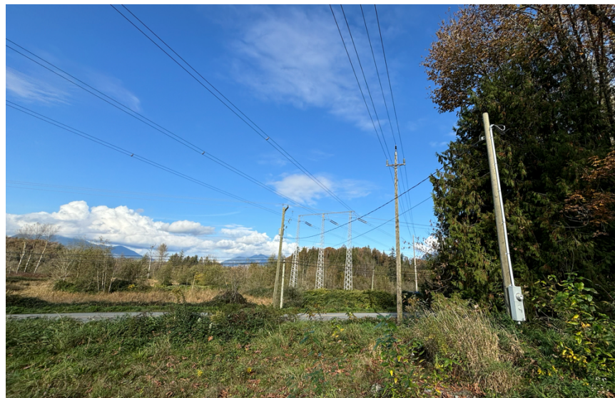
Figure 6: On-site visit photograph of hydro corridor.
