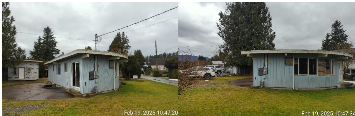
Figures 1 and 2: Photos of existing structure. February 19, 2025.
