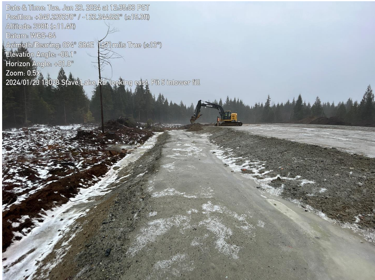
FIGURE 1 LOWER BENCH OF IMPORTED FILL LOOKING TOWARD PIT 5
