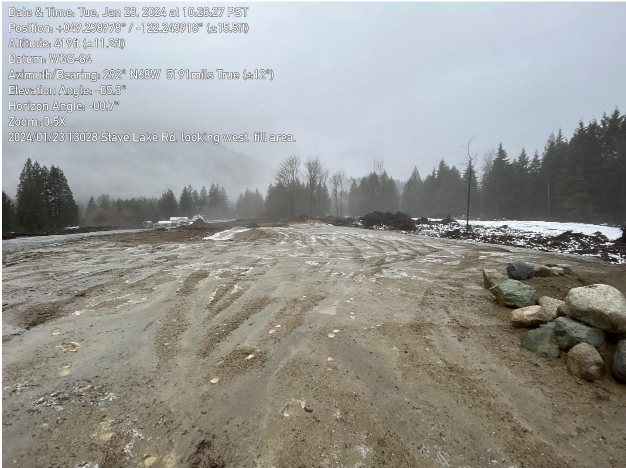
FIGURE 5 IMPORTED FILL (CENTER RIGHT) FROM THE TURNAROUND LOOKING WEST
