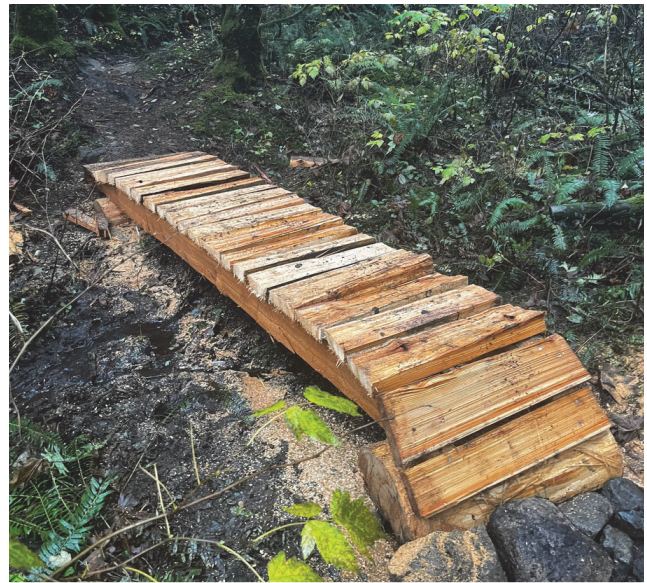
Bridge 14: Replacement. The span of the bridge was extended 2' to put footings beyond the wet areas. Stringers were increased from 3" round to 4x10 milled beams.
