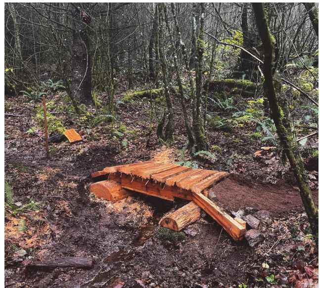
Bridge 16: Was too small for creek when ground water is high. Rebuilt to high water level. Also now further off the ground to prevent build up of debris underneath.
