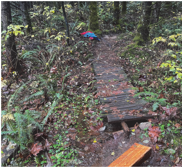
Bridge 14: Prior to replacing. Ground water was seeping out below the footings of the bridge. Stringers were badly undersized (3" in diameter), and rungs had broken off, leaving nails exposed.
