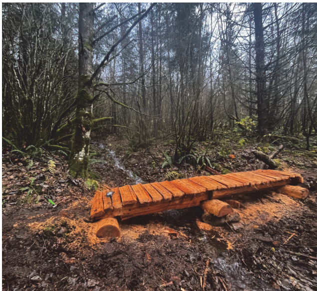
Bridge 15: Built in two spans, for a total of 16'. The original was constructed the same way, but with undersized stringers. Rungs were coming off and were placed too close together allowing water to run over the bridge, further accelerating the deterioration of the bridge. The new bridge is further off the ground to prevent build up of debris under the trail. The mid footing is built up on a foot of rock to keep it out of the water.
