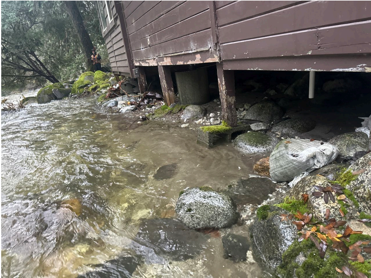
Photo D-19 Looking downstream along the right (south) bank of Emory Creek. Note the cabin footings within the creek. Photo taken by BGC on November 14, 2024.
