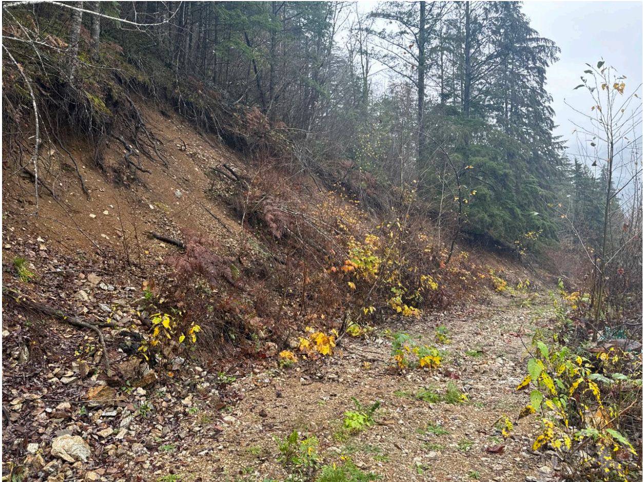
Photo D-28 Looking north at a debris slide along a roadcut and upslope of a home on Baker Road. Photo taken by BGC on November 14, 2024.
