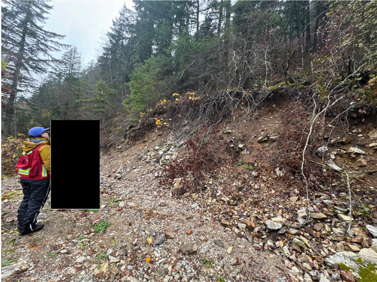
Photo D-29 Looking upslope at a debris slide along a roadcut above a house on Baker Road. Photo taken by BGC on November 14, 2024.
