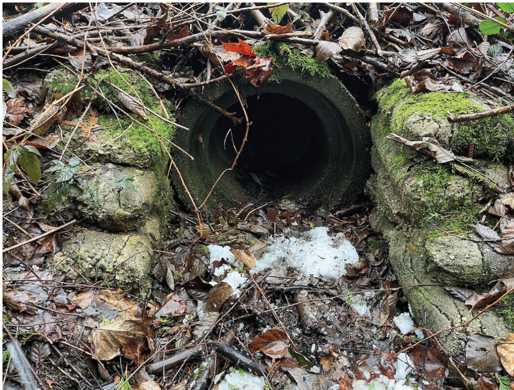
Photo 17: January 23, 2024. Looking at the inlet of the 450 mm diameter concrete culvert as part of the Dewdney Dike floodbox. The inlet is at El. 6.35 m and is adjacent to the southwest corner of the Subject Property which is the lowest point on the Site.
