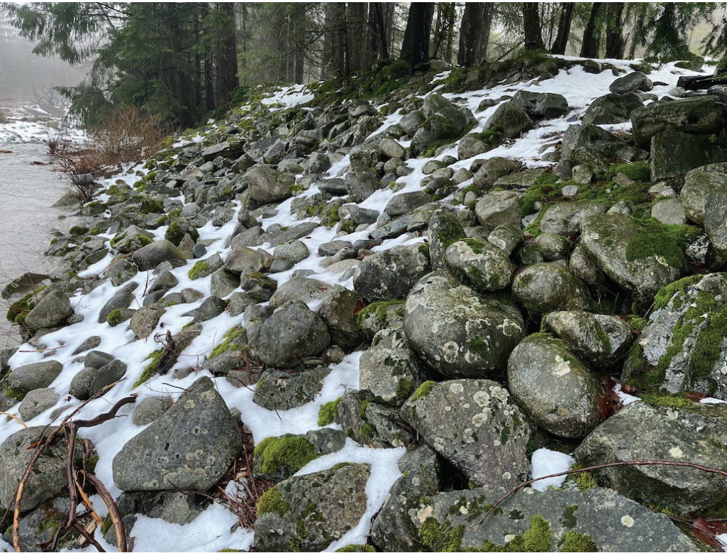
Photo 27: January 23, 2024. Looking south (downstream) on Norrish Creek at the upstream end of the armoured right bank river dike near the fan apex.
