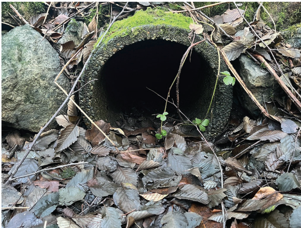
Photo 20: December 15, 2023. Looking at the outlet of the 450 mm diameter concrete culvert as part of the Dewdney Dike floodbox. The outlet is on the west side of the dike.
