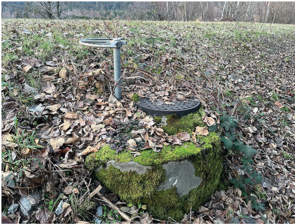
Photo 19: December 15, 2023. Looking at the floodbox manhole cover and wheel on the Dewdney Dike adjacent to the southwest corner of the Subject Property.
