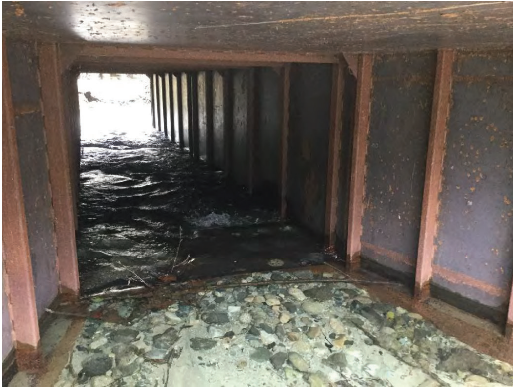
Photo 21: March 28, 2018. Looking downstream on Inch Creek at the inlet of the steel box culvert under the CP Railway. The culvert has a span of 2000 mm and a rise of 1600 mm (SGL 2018).
