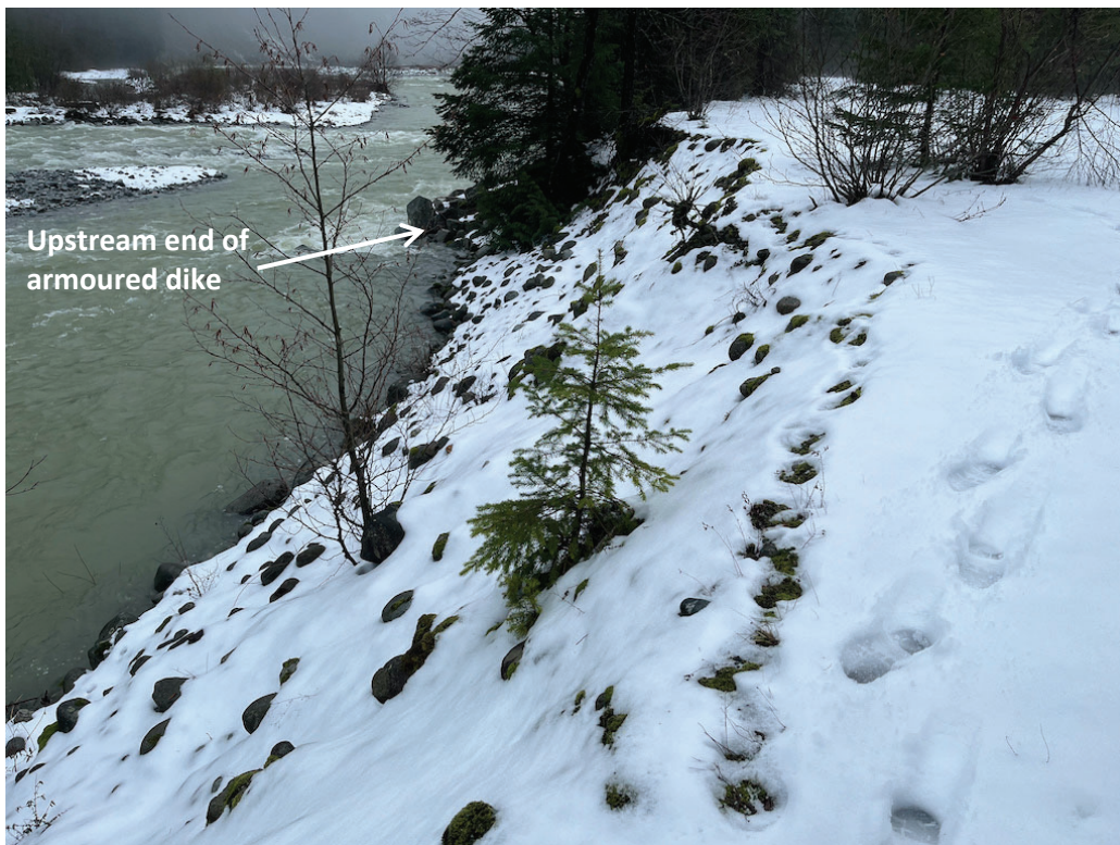
Photo 30: January 23, 2024. Looking south (downstream) on Norrish Creek at the eroding right bank upstream of the dike near the fan apex. The upstream end of the armoured river dike is in the background.
