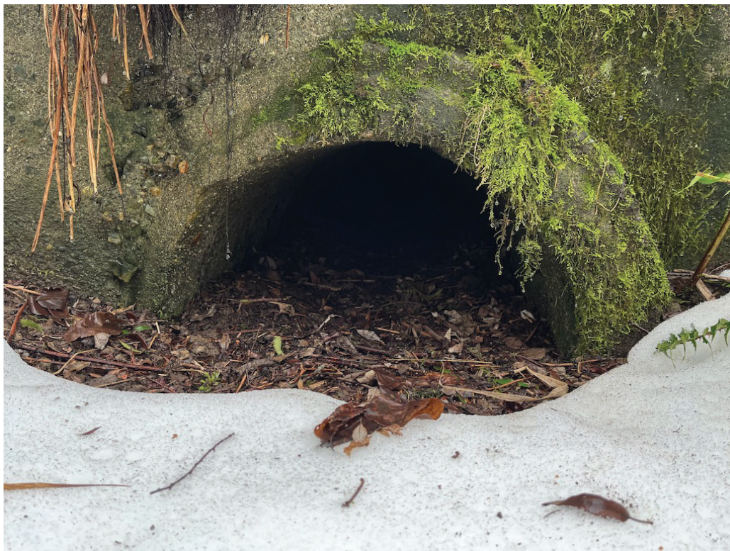
Photo 22: January 23, 2024. Looking at the outlet of the 600 mm concrete culvert located under the CP Railway adjacent to the middle of the Subject Property. This culvert does not convey flow, there is no defined channel, and the inlet is buried and could not be located.
