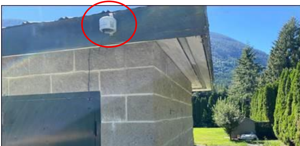
Figure 1. A Purple Air sensor installed in Electoral Area E to measure local concentrations of fine particulate matter.
