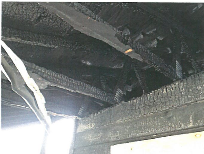
Photo 5: Roof and Wall damage over back deck/walkway
